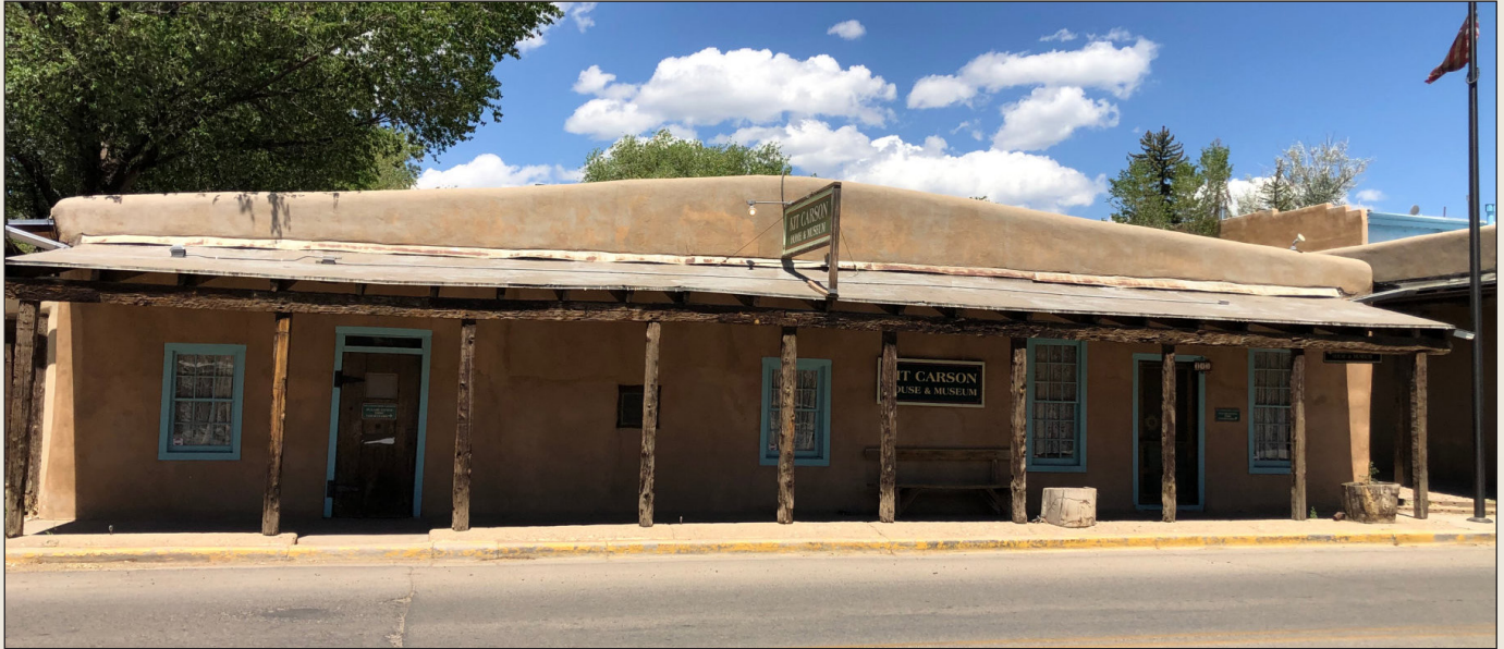
Kit Carson House front elevation photo by Roy Woods
